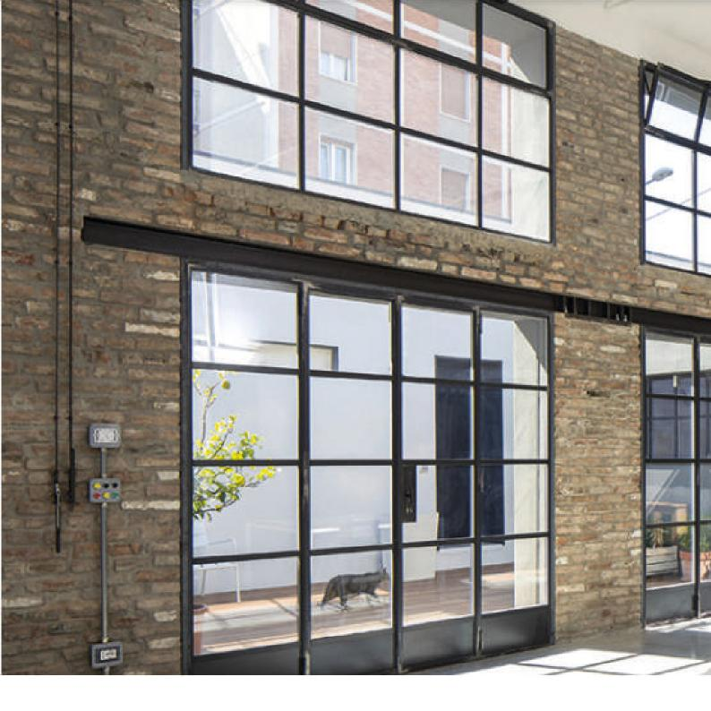
External steel windows and doors has been in production for decades and has proven itself with durability and endless design options while keeping the characteristic appearance to any project which requires a visual link to historical hot rolled steel profiles.
